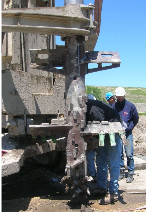
Figure 145. Photo. Second view of typical tools used for WRE mixing.
