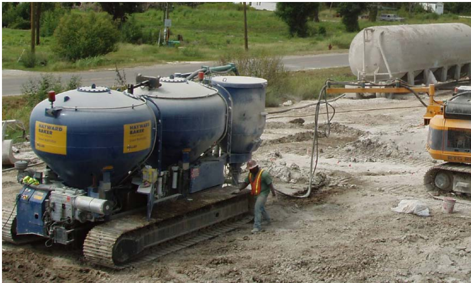
Figure 150. Photo. Typical binder delivery unit for dry mixing.
