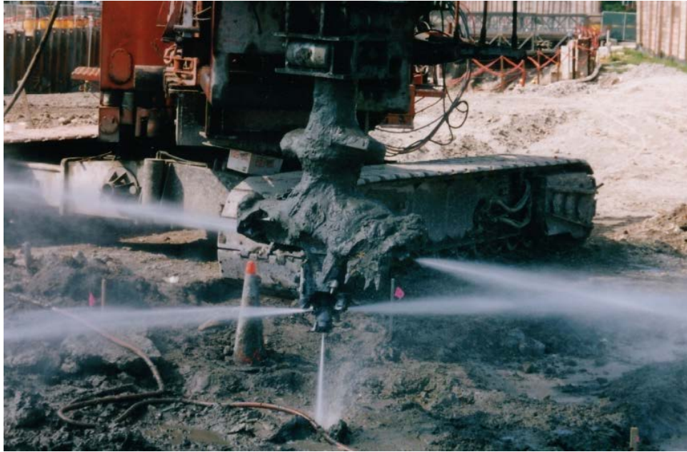
Figure 147. Photo. Example of a WJE tool. (127)
