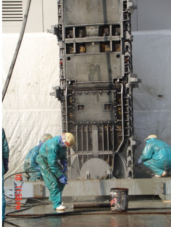
Figure 148. Photo. TRD tooling.
