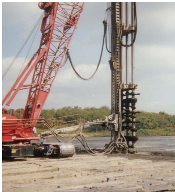
Figure 141. Photo. Second view of typical blade-based tooling for WRS mixing. (127)
