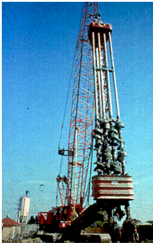
Figure 139. Photo. Typical WRS mixing machine.
